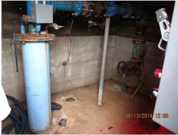
The pumps and electrical boxes of Oakville's water pump station have been elevated several feet, providing protection up to the 2007 flood.
