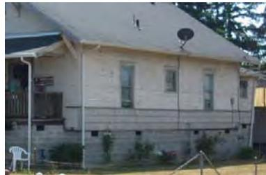
This is an example of an improperly elevated building in the Basin. The openings are too high to relieve hydrostatic pressure.
