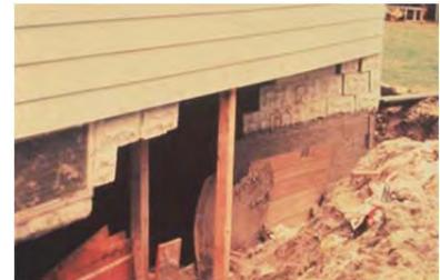
This is what happens to a block wall when the openings do not meet code and water pressure is not equalized.
