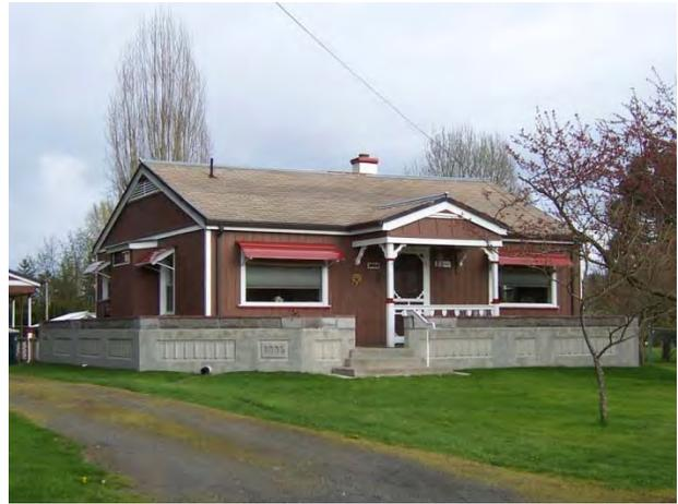
The owner of this house in Centralia built this floodwall around the house after his first flood. It has worked during subsequent floods.
