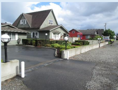
Local flood wall
