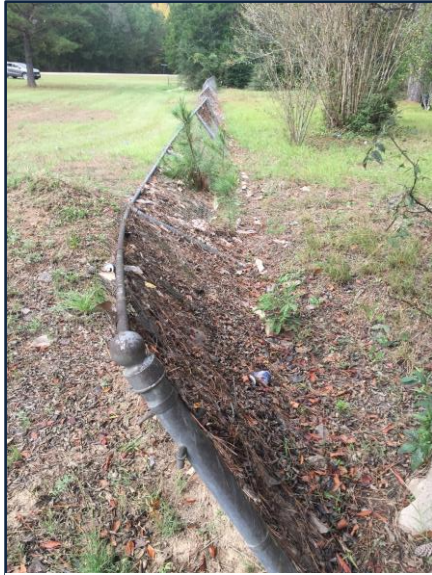
Figure 1: An example of how a chain link fence becomes a debris dam.
