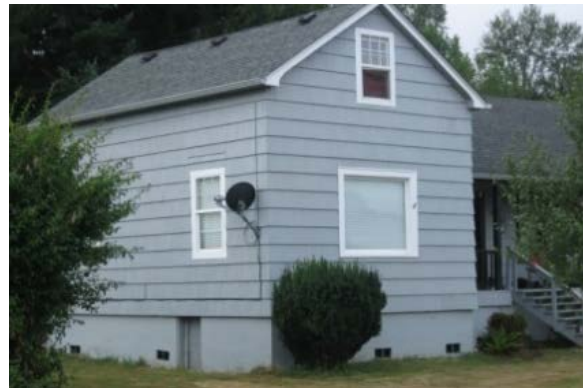
This is an example of a properly elevated house. Note the location of the openings, near the ground.
