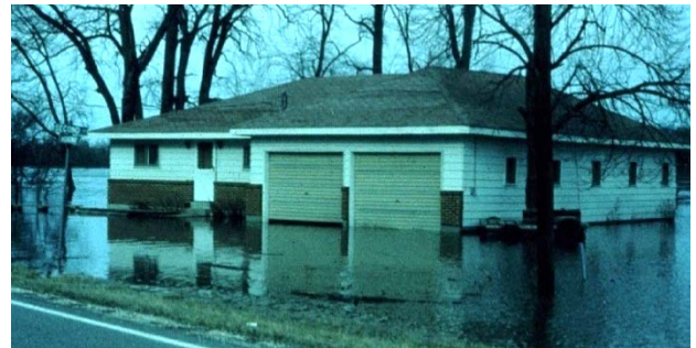
Before, During, and After Elevating a House
