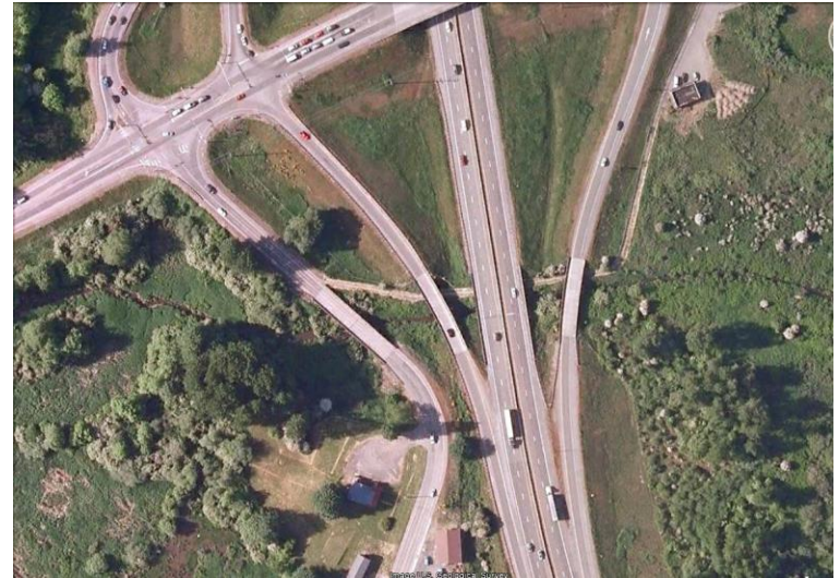
I-5 crossing of Dillenbaugh Creek
