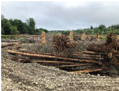
Engineered log jams (shown above) are an important habitat component for the EF Satsop River Restoration Project.
