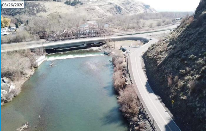
Nelson Diversion Dam on Naches River
