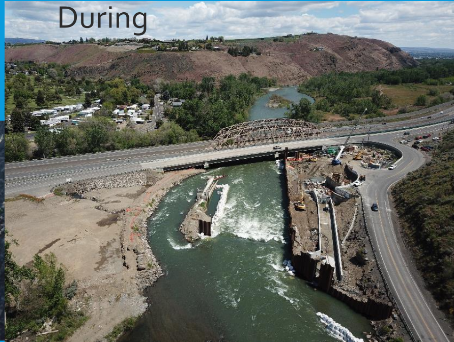
Nelson Diversion Dam during construction
